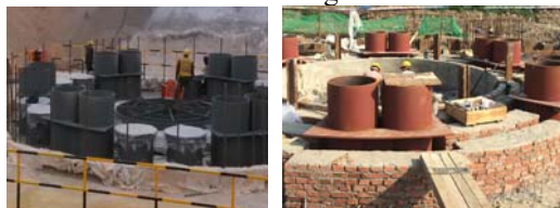
Fig.4: Construction situation of traditional method and present method
