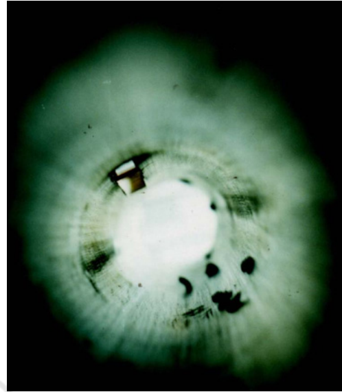
Figure 5: View from the robot's camera inside the pipeline.
